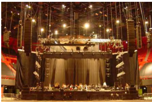
Figure 74: Hybrid flown/stacked subwoofer example : L/R = 14 V-DOSC + 3 dV-DOSC (per side); flown dV-SUB (6 per side); ground stacked SB218 (6 per side); LL/RR = 4 V-DOSC + 6 dV-DOSC (per side); stereo infill = 2 dV-DOSC (per side); distributed front fill = 4 dV-DOSC (Bjork, POPB Paris 2003 – sound design M Malki)
