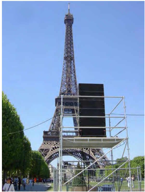
Figure 88: Flown and stacked delay systems (sound design - D. Tramontani, A. Francais, resp.)
